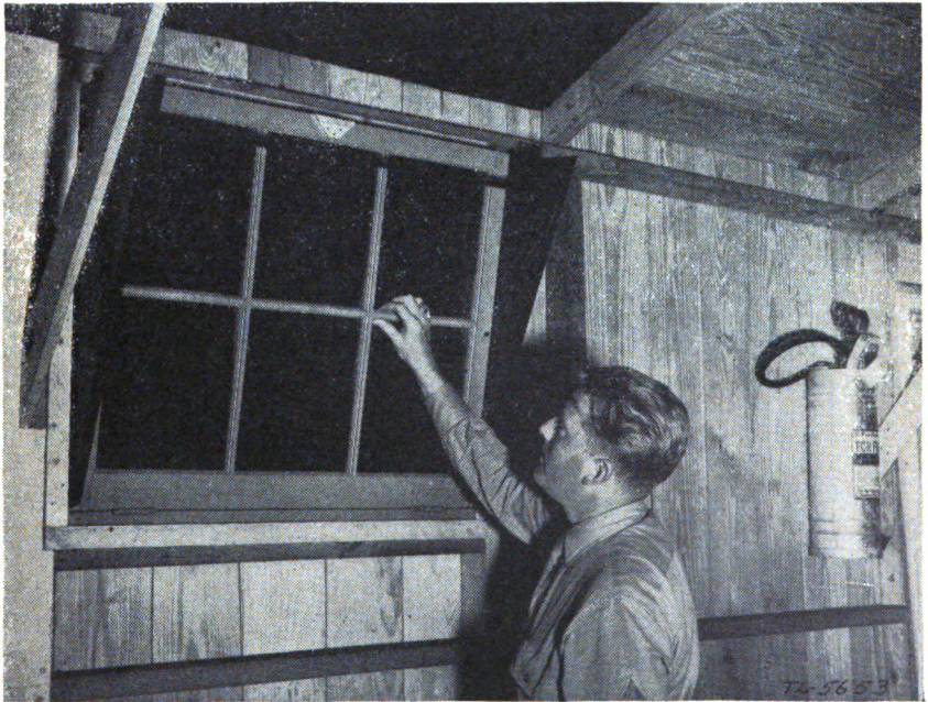
FIGURE 42.—Painted windows with ventilation blinders.
