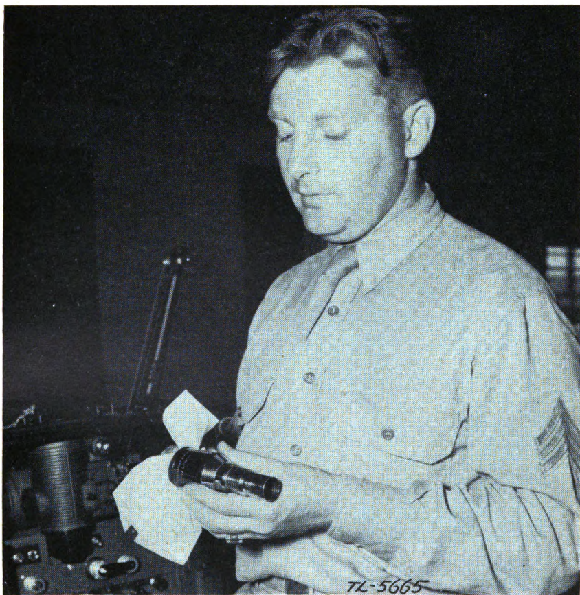
FIGURE 53.—Cleaning lens with tissue.
